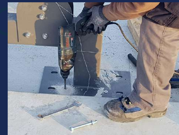
Plates for concrete plinth
